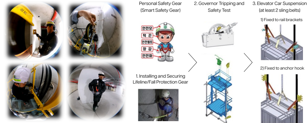
MRL Expansion Type 3+1 (Wearing Safety Gear/Lifeline Installation/Governor Operation/Car Suspension)
