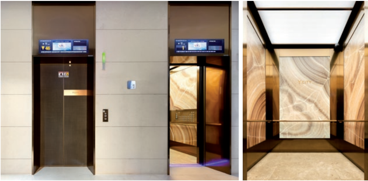
Ilsan Y-CITY Sixty-six elevators were installed, including twenty-four 4 m/s units and six 3.5 m/s units, as well as twenty escalators.
