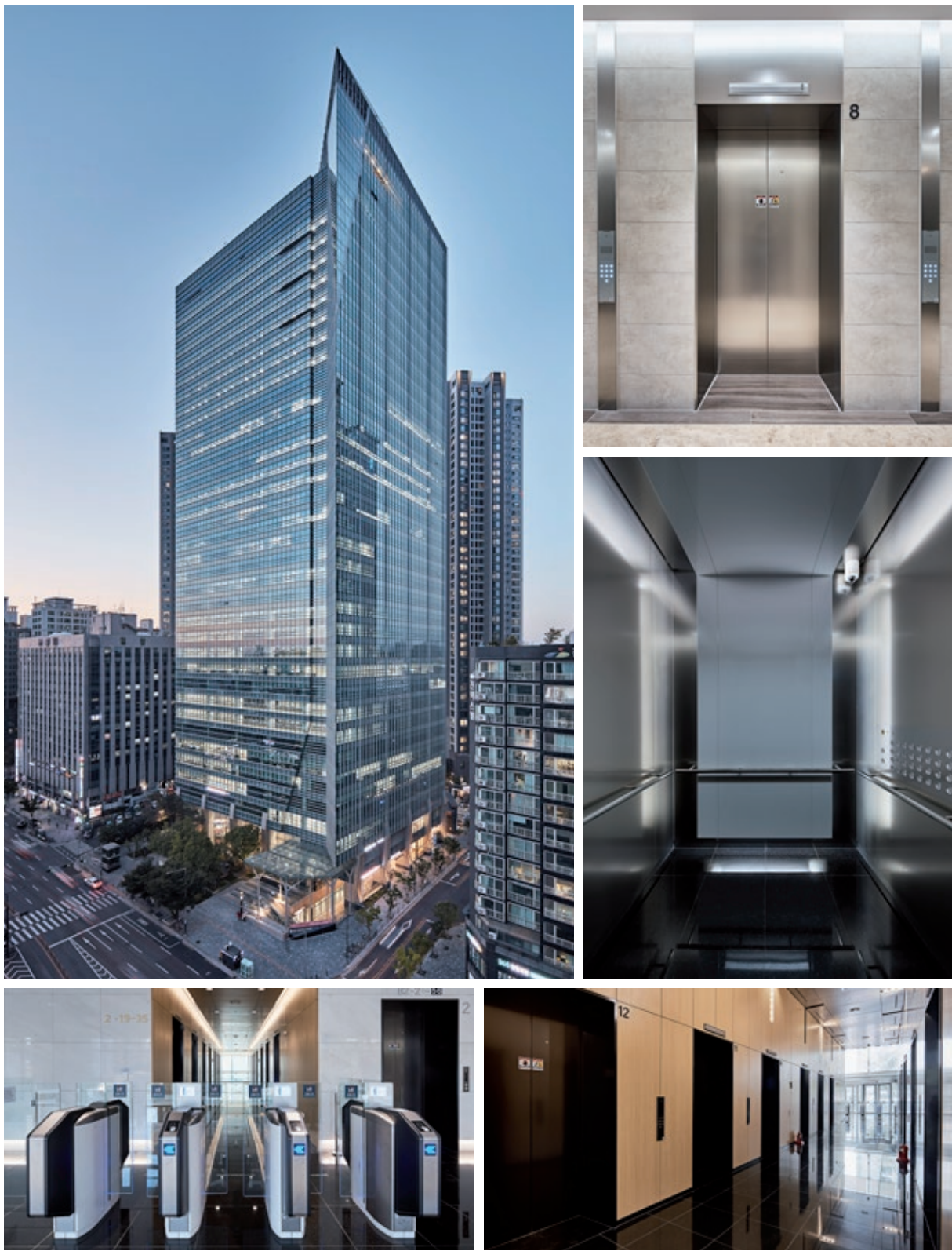
East Central Tower Eighteen elevators were installed, including thirteen 4 m/s units, as well as five escalators.
