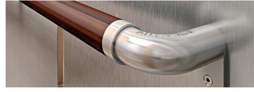
Hyundai Elevator's antiviral handrails eliminate more than 99% of harmful bacteria. This is done by applying antiviral materials to the handrails inside elevator cars, preventing the transmission of harmful substances often found on them.
