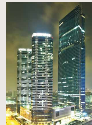
Hanoi Landmark Tower (72 FL.) Hanoi, Vietnam Speed : 240m/min (2units), 210m/min (10units) Total : 29units
